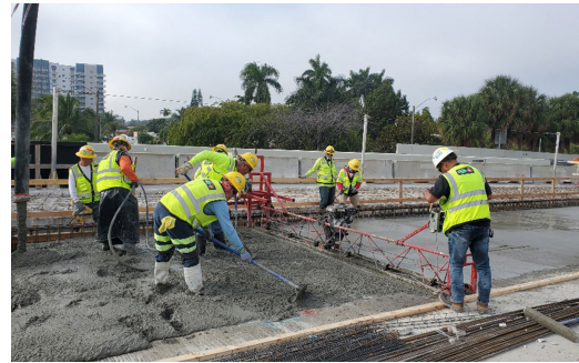
Concrete roadway deck pour for bridge widening on SR 836.
