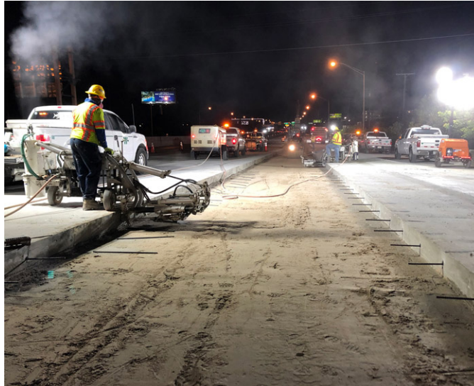
Crews preparing for concrete pavement replacement on I-95
