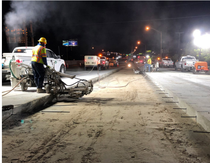
Crews preparing for concrete pavement replacement on I-95
