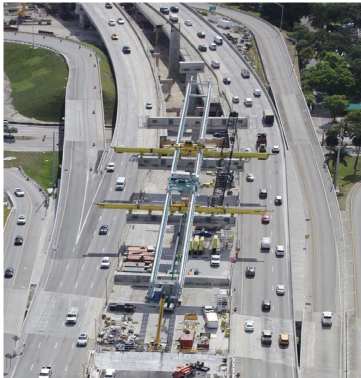
SR 836 bridge cap and beam lifter just west of NW 17 Avenue
