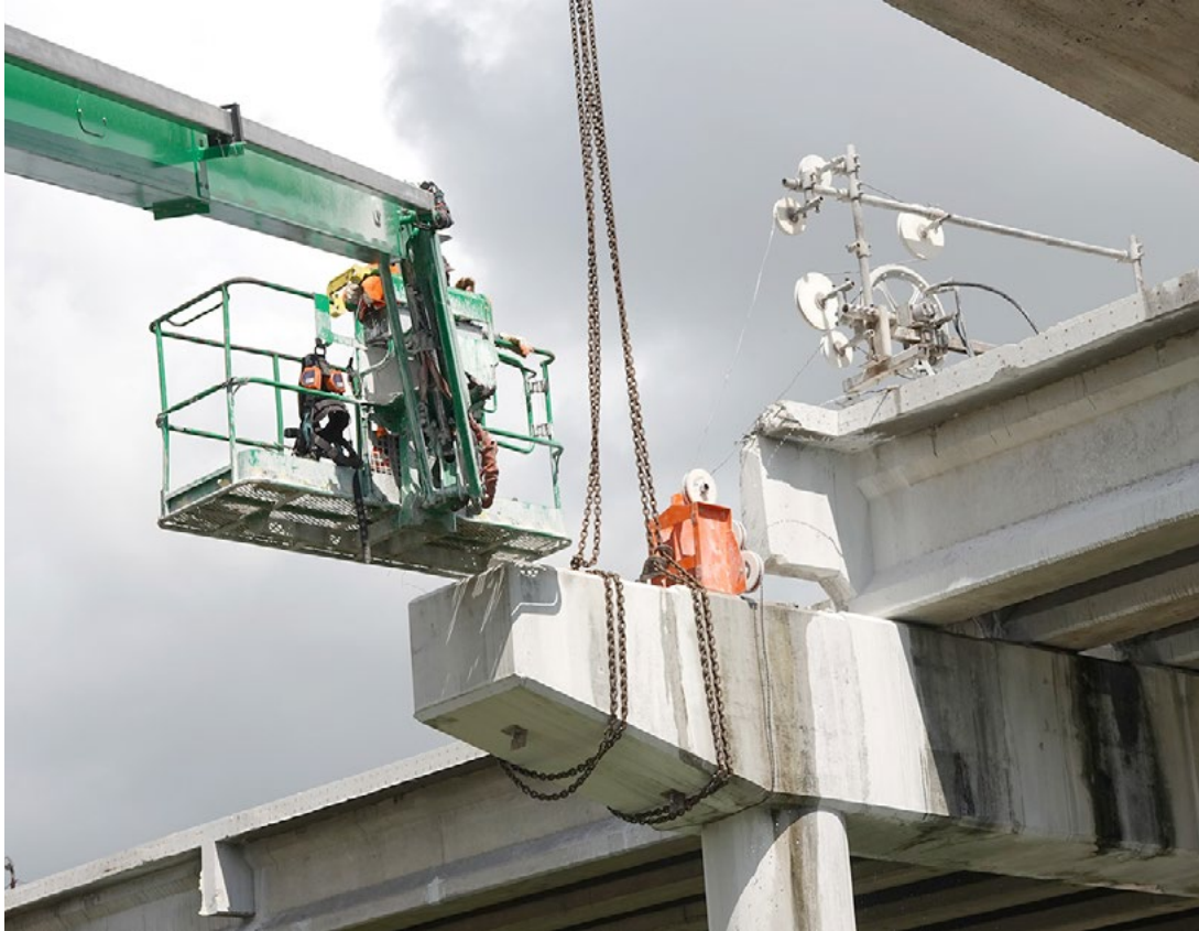
Concrete cutting operations at SR 836 near the core of the interchange
