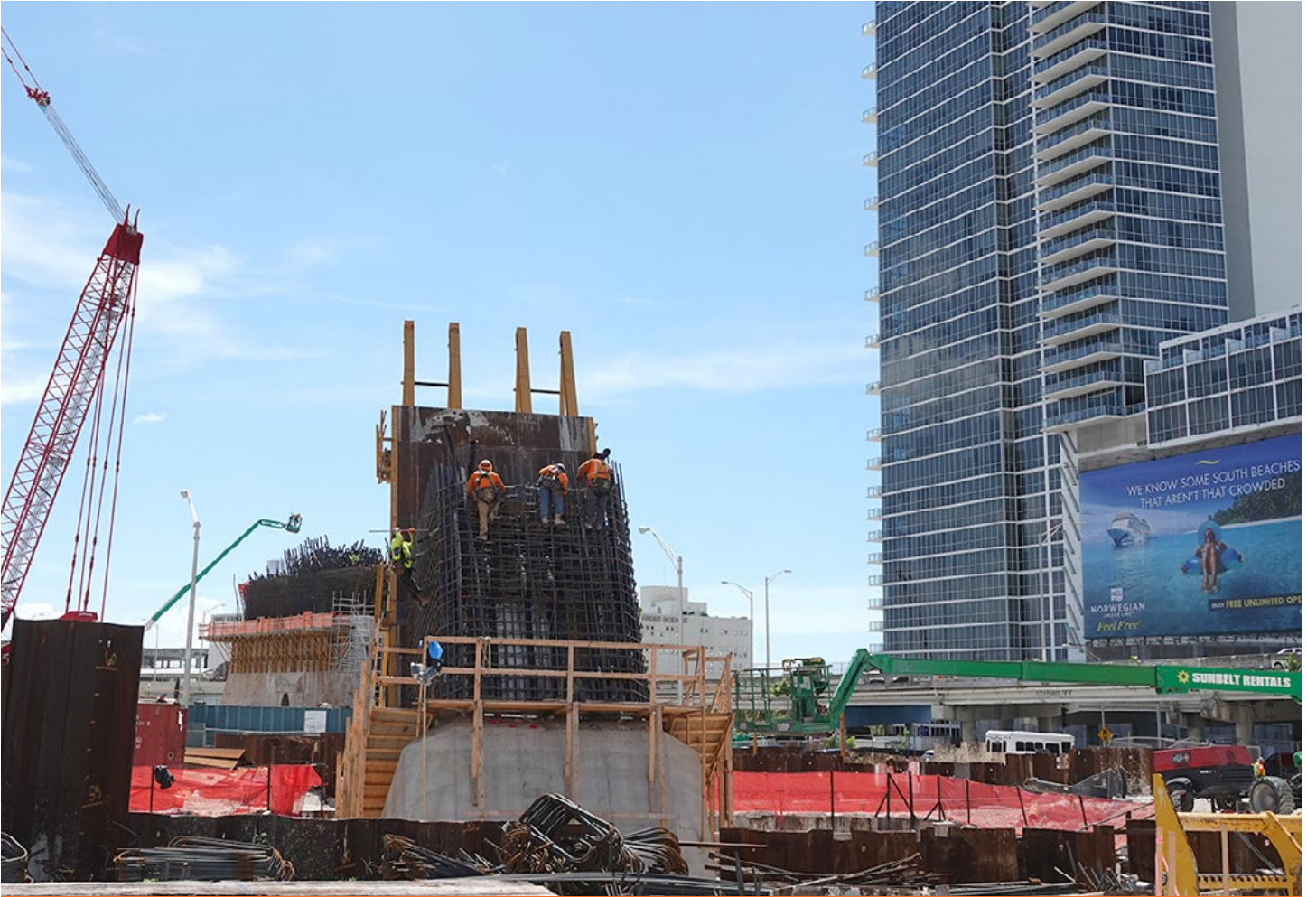
Crews installing reinforcing steel at one of the signature bridge arches
