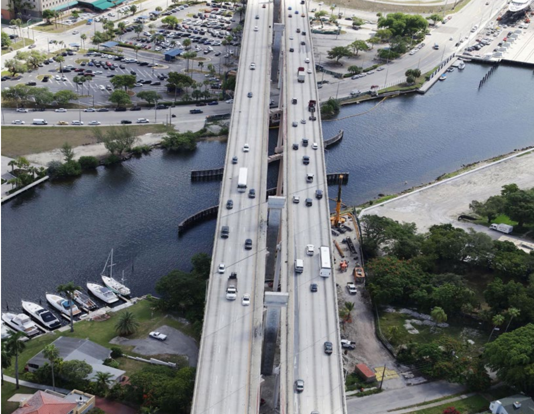
Completed piers on both sides of the Miami River
