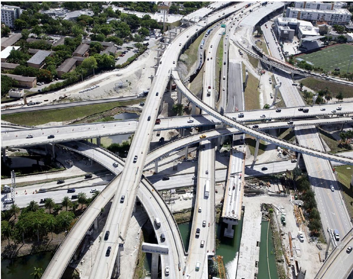
Ongoing construction at the SR 836/I-95/I-395 interchange core
