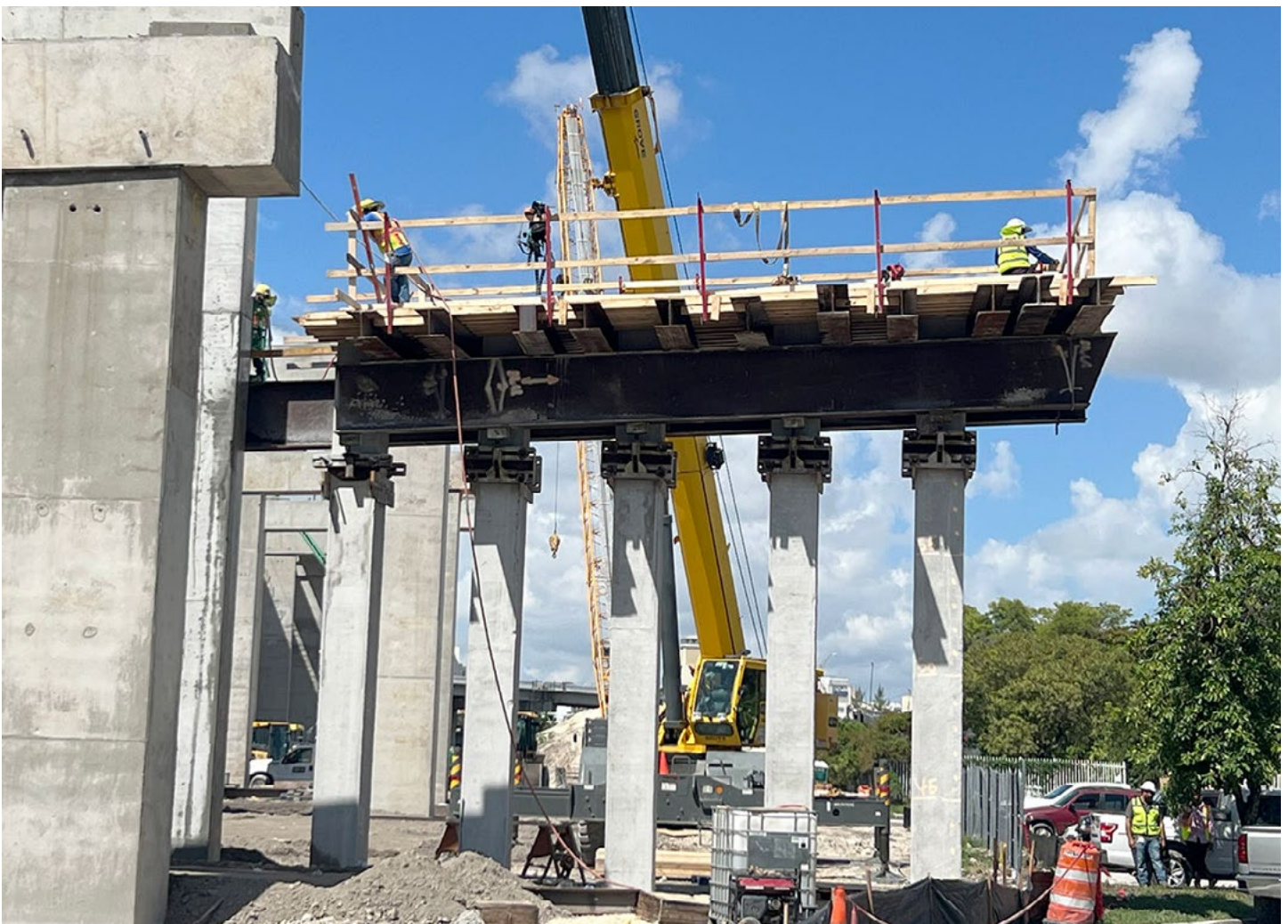
Work on a bridge cap for I-395 just east of I-95
