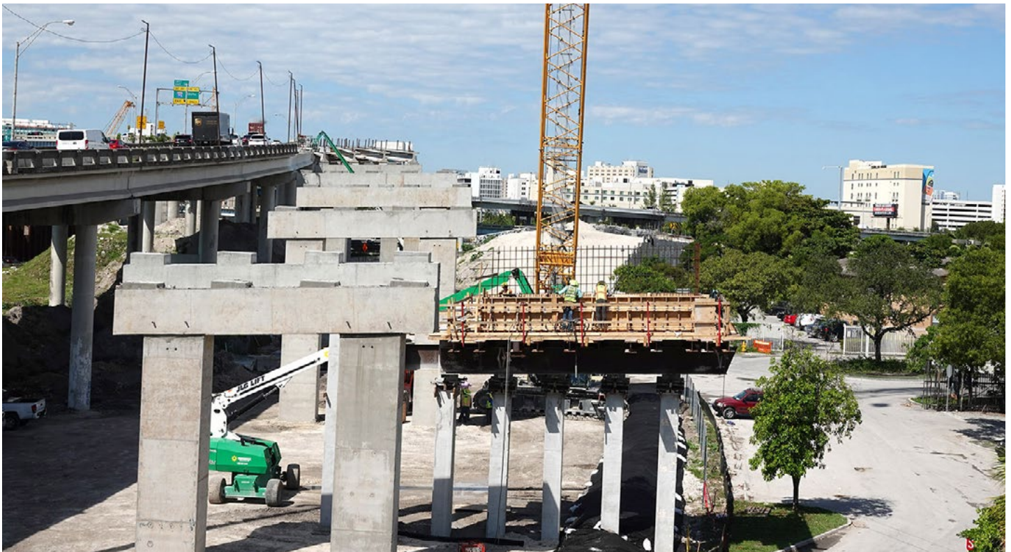
Bridge cap construction on I-395 just west of NW 4 Avenue
