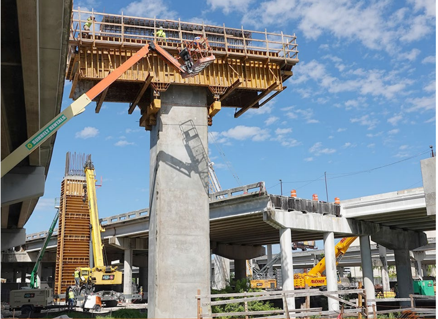
Pier cap construction at the core of the interchange
