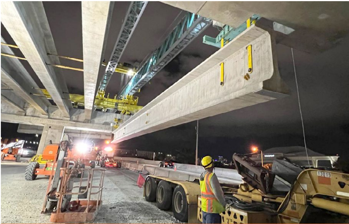
Ongoing installation of SR 836 bridge beams just west of NW 17 Avenue.
