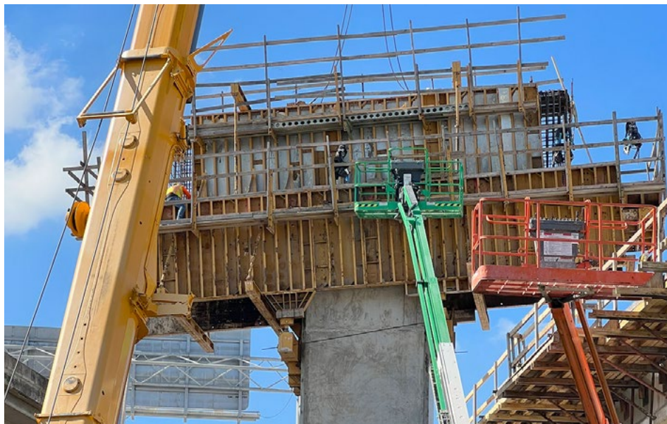
Pier cap construction at the core of the SR 836/I-95/I-395 interchange
